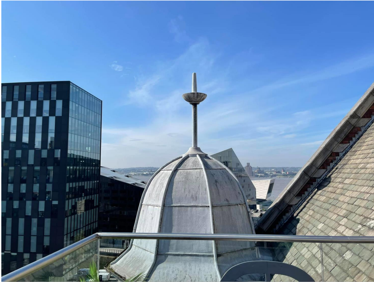
Views from the balcony.
