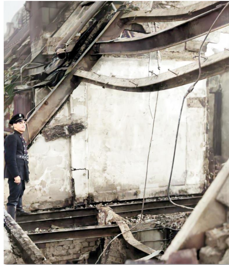
The bombed remains of 30 James Street showing the turret top to the left. Above shows the sagging of the roof beams high up in the attic space of the building. Please note these images are copyright Historic England.
