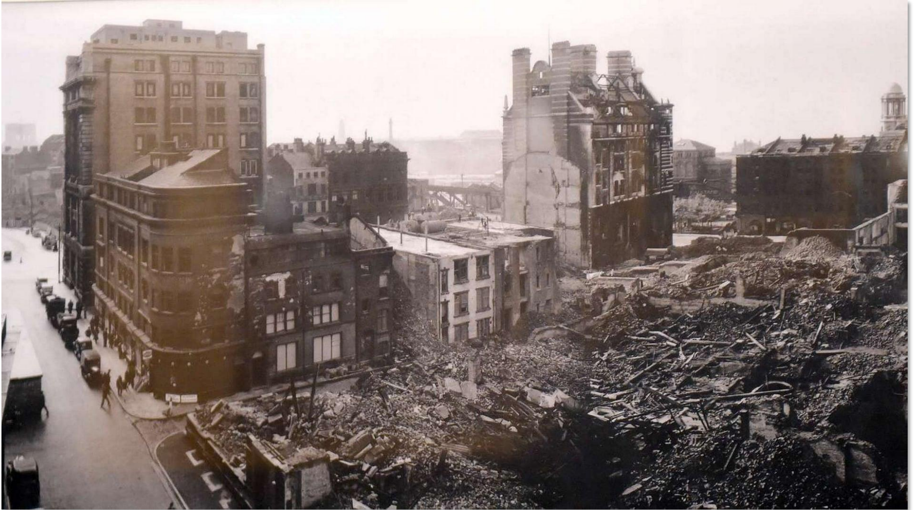
Viewing the rear of 30 James Street – a burnt out shell.
