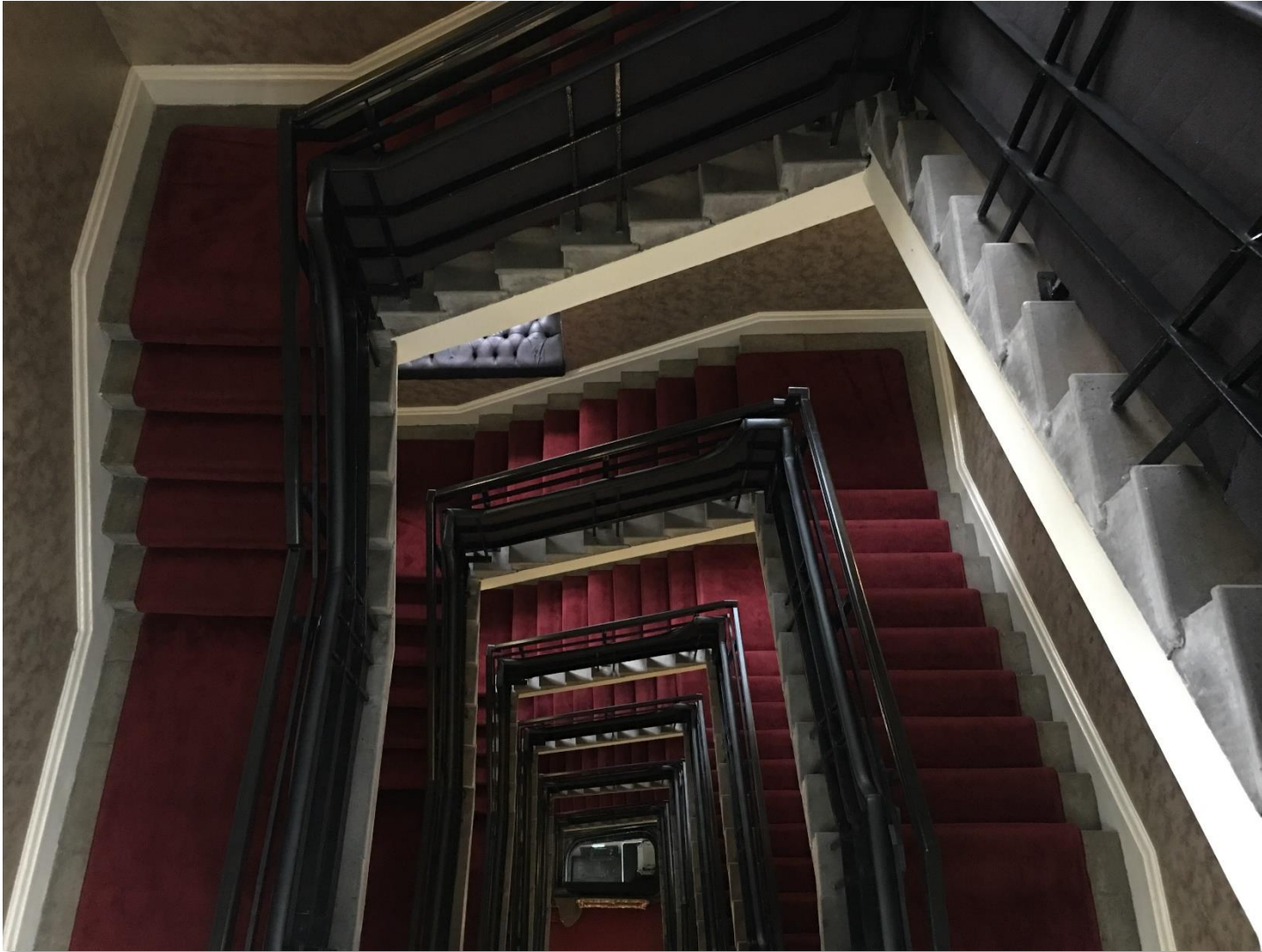
Looking down from the top of the staircase.
