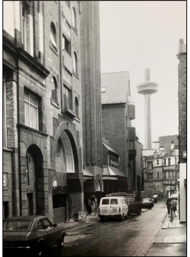
Above is the newly constructed Cavern Walks, taken from Dorans Lane and Harrington Street, 1984. Copyright Liverpool City Council
